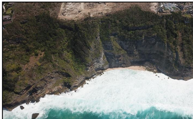
Figure 3. The 150-meter tall, almost vertical cliff face at Site B, with slight recess at the lower part.
